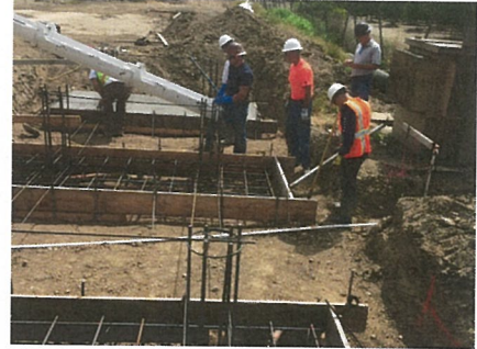
New Concrete Foundations being placed by Contractor
