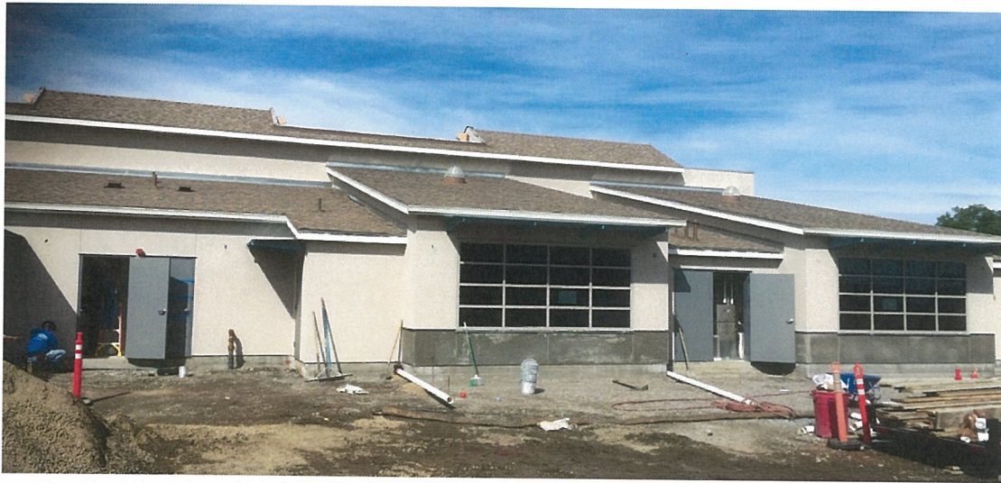
Progress Photo of the New Classroom Building
