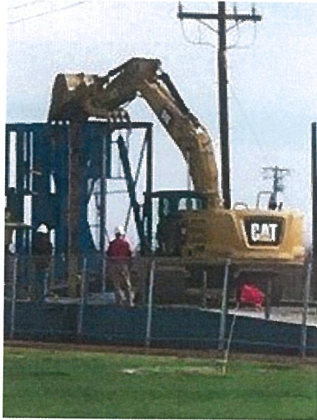
Demolition of old press box
